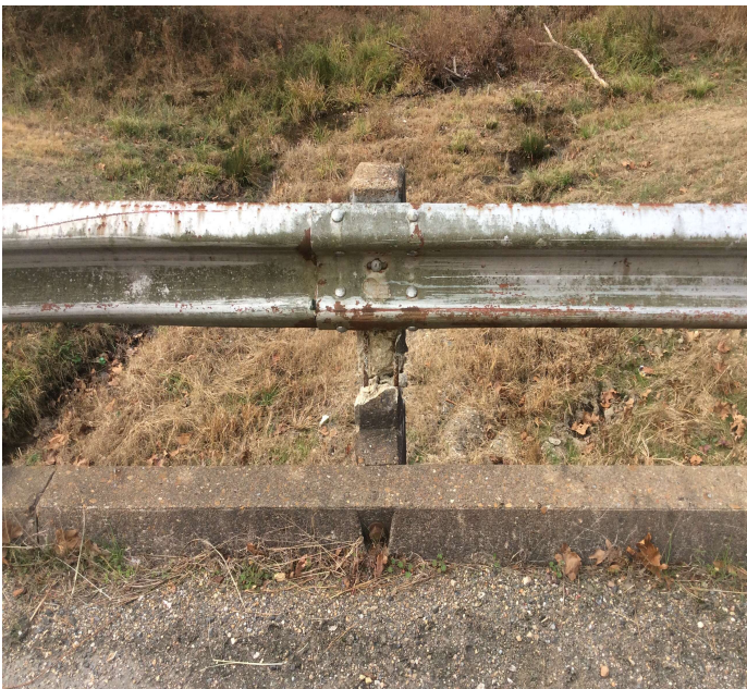
PHOTO 1 Description 4th rail post on the left side is broken and rail is bent.
